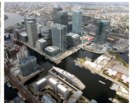
Modern Canary Wharf
